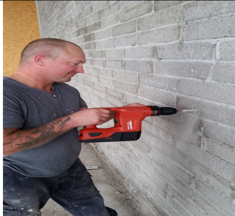
Poor practice – Using Hand-held drill with no on-tool extraction (David Flynn Ltd, IE)
